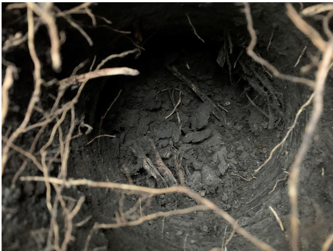
Photo 23: Showing inside borehole BH8 sampling location (0.5-0.6m) at 3 Holdsworth Avenue, St Leonards.
