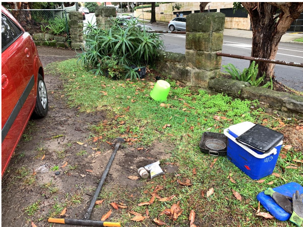
Photo 16: Showing borehole BH4 sampling location at 10 Marshall Avenue, St Leonards.
