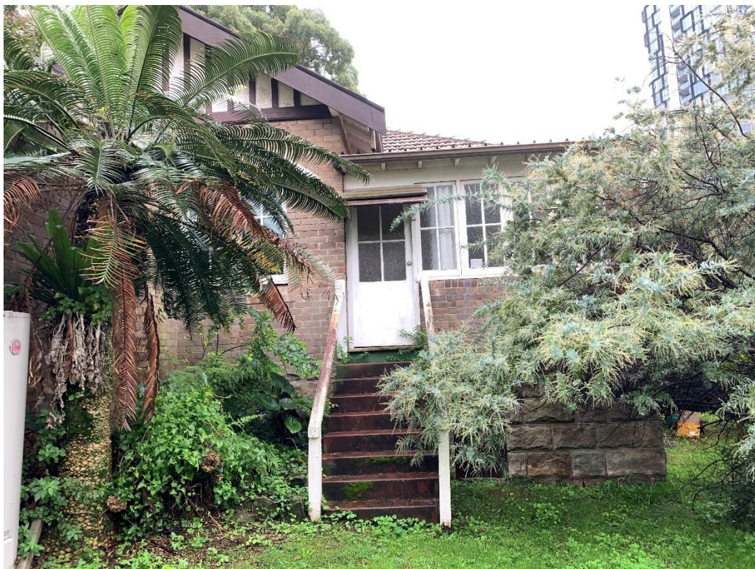
Photo 14: Showing the rear of 10 Marshall Avenue, St Leonards, looking north.
