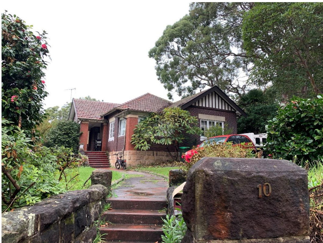
Photo 13: Showing 10 Marshall Avenue, St Leonards, looking south.
